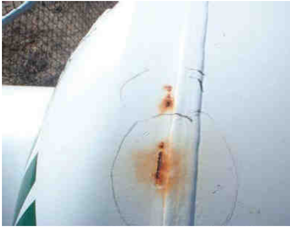
Figure 12.3 Surface rust surrounding a tank weld
