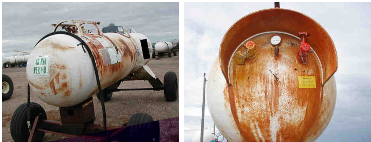
Figure W13: Examples of rusted tanks in need of potential repair and repainting.
