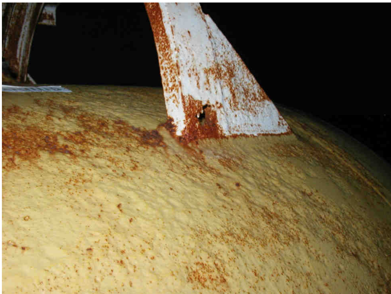
Figure W14: Example of severe corrosion due to years of bad paint and leaking valves.
