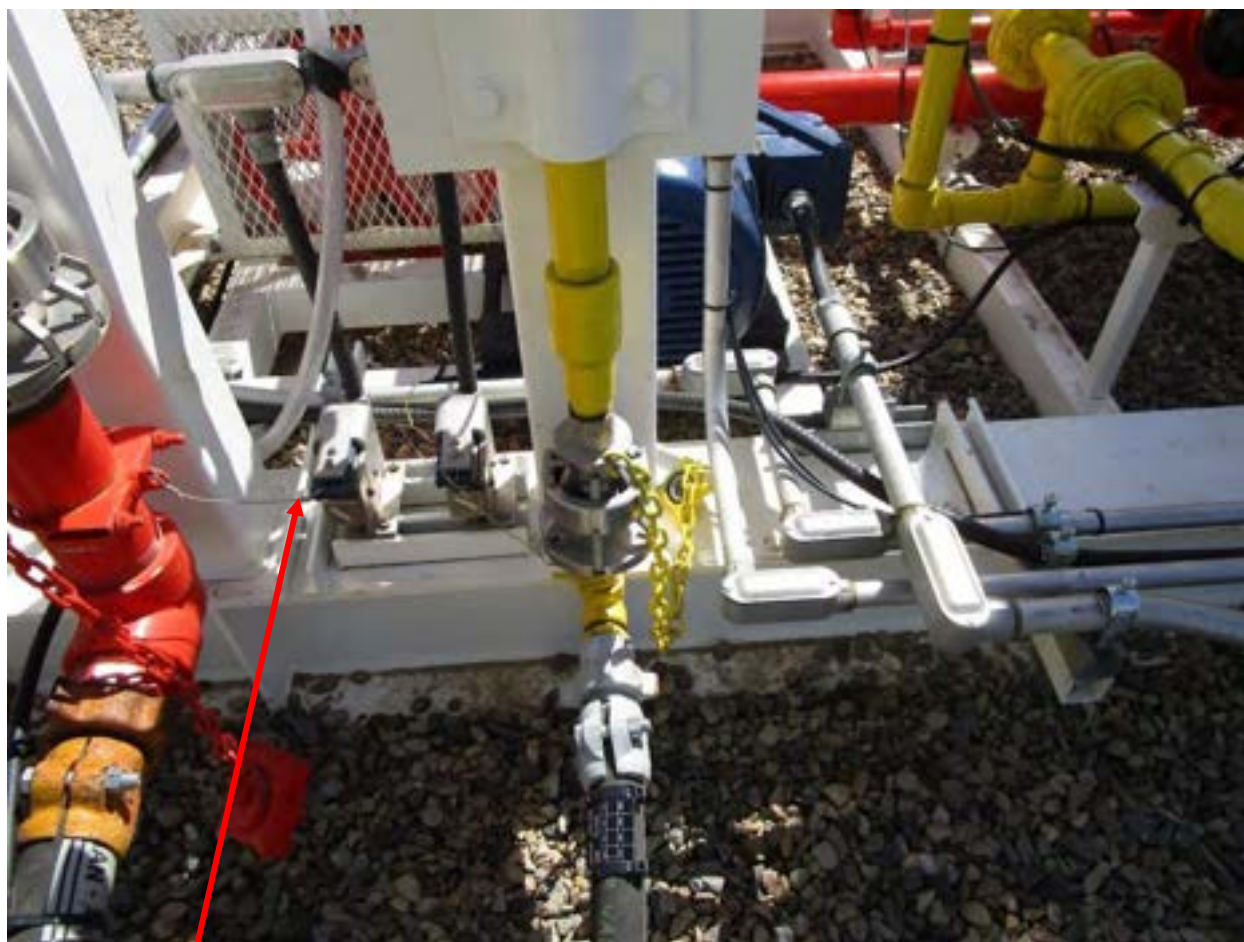
Cables connected to electronic shut down
