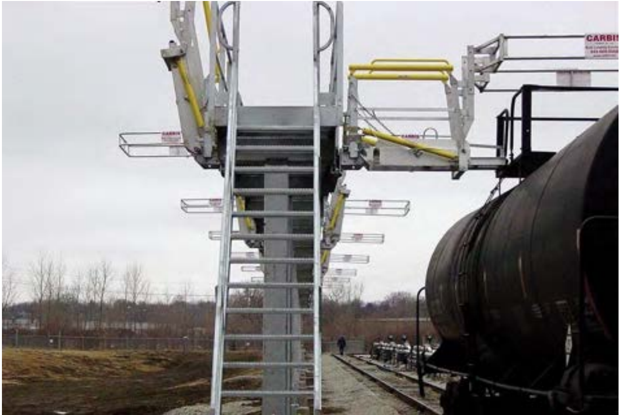
Figure 5. Example Fall Restraint System
