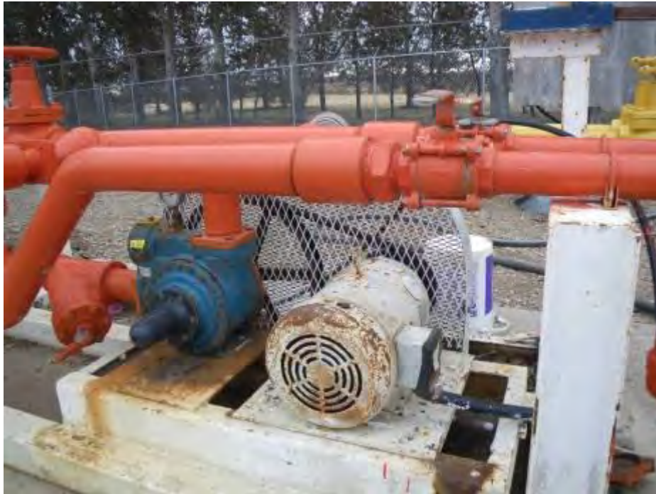
Figure 12. Guards on Transfer Pumps/Compressors – Example 1
