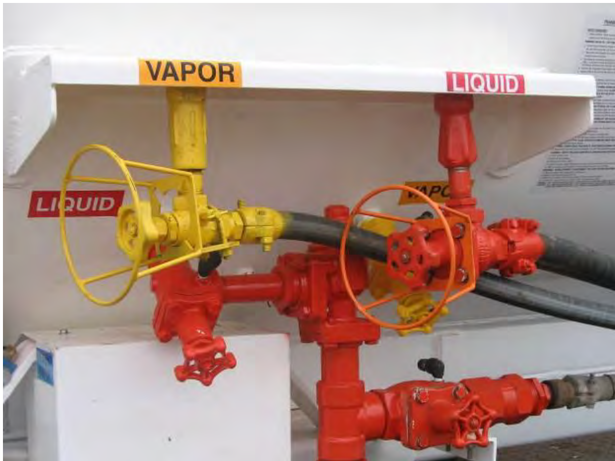
Figure 4. Typical hose end valve protectors.
